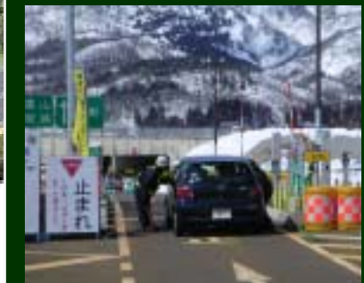
Ingress lane of Smart Interchange
