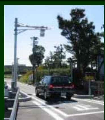
Egress lane of Smart Interchange
