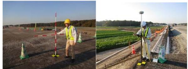
Fig.4 GCP Measurement by VRS-GNSS Surveying
