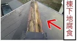
棟下地腐食  |
