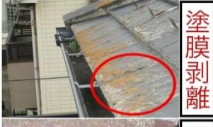
塗膜剥離 |
