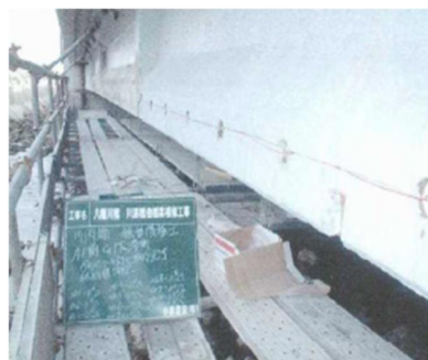
写真-4 犠牲陽極設置状況
