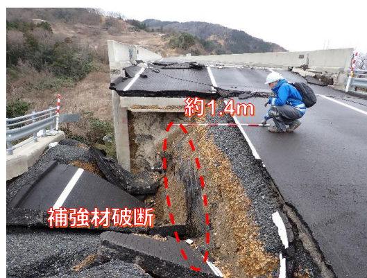
(c)補強材の状態
