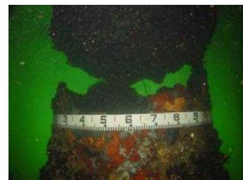
栈橋杭の破断
