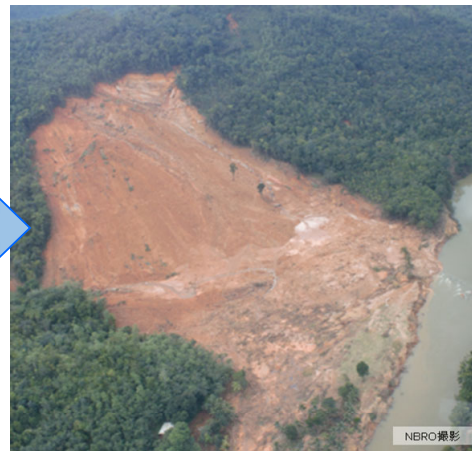
(Right) Large-scale failure confirmed at the site.
