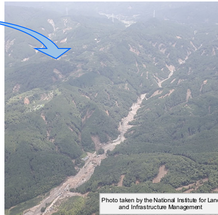
(Right) Area where failure occurred frequently that was identified by the
