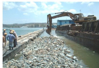
Figure 4-14 Concrete block fabrication (left), installation (center), and stone backfilling (right) at Sihanoukville Port
