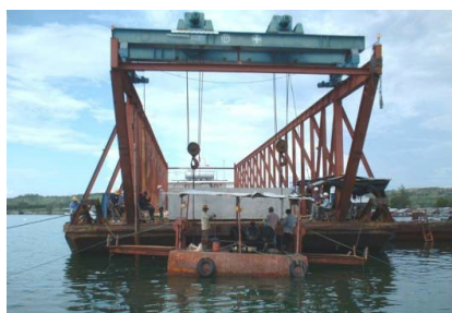
Figure 4-14 Concrete block fabrication (left), installation (center), and stone backfilling (right) at Sihanoukville Port
