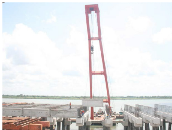
Figure 4-13 Steel pipe pile quaywall construction at Phnom Penh Port (river port)
