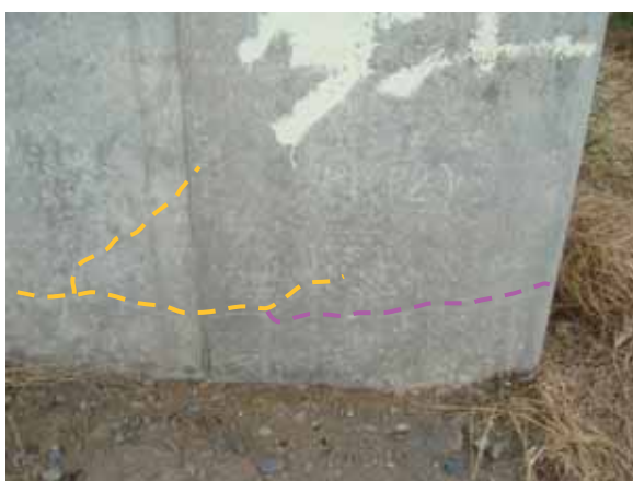
(a) P1 橋脚
