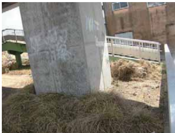
(a) P1 橋脚
