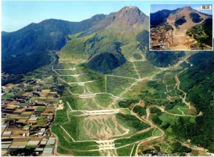
Fig. 1: Image of the completed sediment control facilities on the Mizunashi River of Unzen and Fugendake
