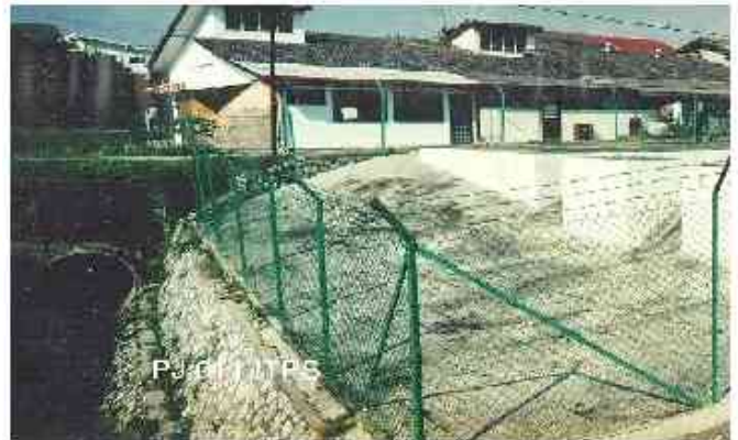
Figure 10: Communal Septic Tanks
