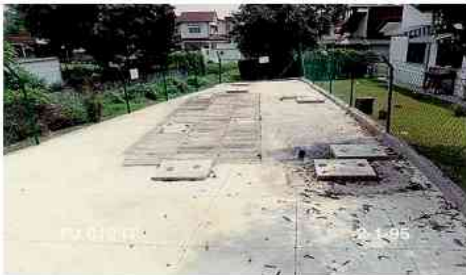
Figure 10: Communal Septic Tanks
