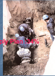
Repairing work of distribution main pipe
