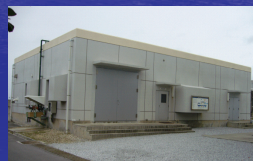
Advanced Wastewater Treatment Plant
