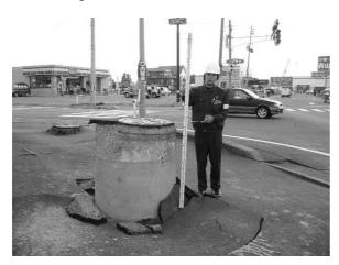
Photo1. A lift-uped manhole in Niigata-ken Chuetsu Earthquake
