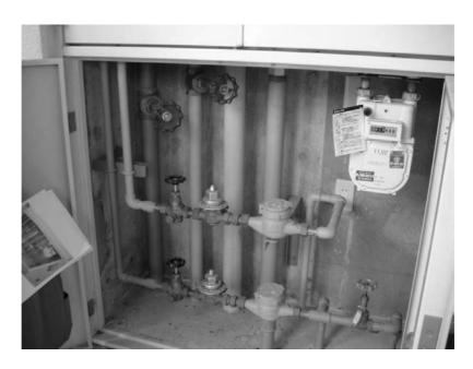
Photo 1 Example of distinction by color-coding the pipes (Yellow is reclaimed wastewater, blue is drinking water)
