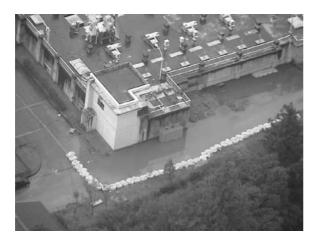
Photo2.A temporary settlement pond and a disinfection plant in Horinouchi Treatment Plant
