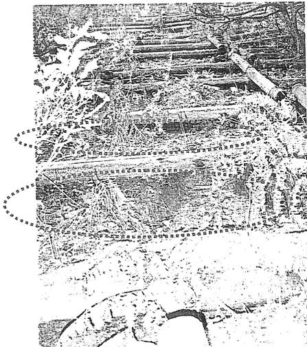
**Tsuchiyabara hillside work:** The surface flow on the slope scours the ground under the thinned material so that is above the ground, allowing the sediment to move. This delays the recovery of the vegetation.
