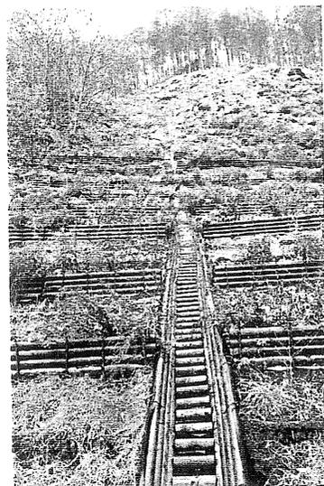
**Nomugi Pass hillside work:** As in the case of the Tsuchiyabara hillside work, thinned material is used to make the foundation work, but the surface and underground water flows are appropriately performed so that no scouring can be seen.
