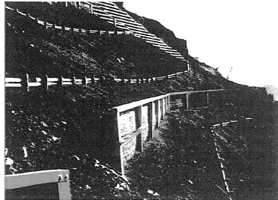
**Onagi hillside work:** on the earth retaining work, scoria that is easily moved by the wind etc. was firmly solidified.
