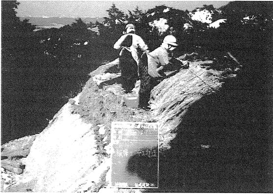
**Tanakami hillside work:** Initially slope surface treatment between seedling terracing work was not done, but because the seedling terracing work was buried by sediment, straw covering was done beginning in 1960. This stabilized of the slope and the trees grew normally.
