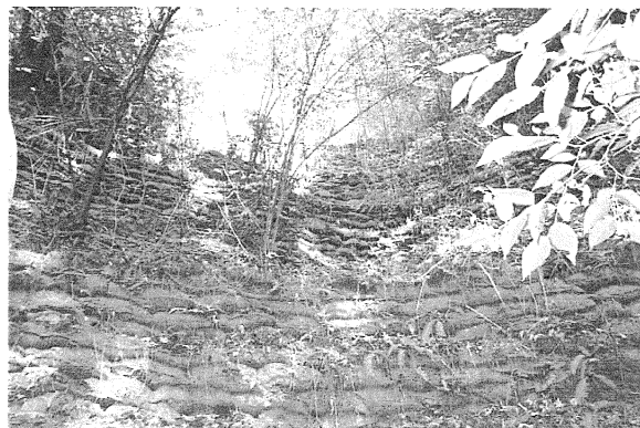
Tsuchiyabara hillside work: Use of bags of soil Professor Ote studied the use of soil cement as material to fill soil bags in the Kyoto University Forest.
