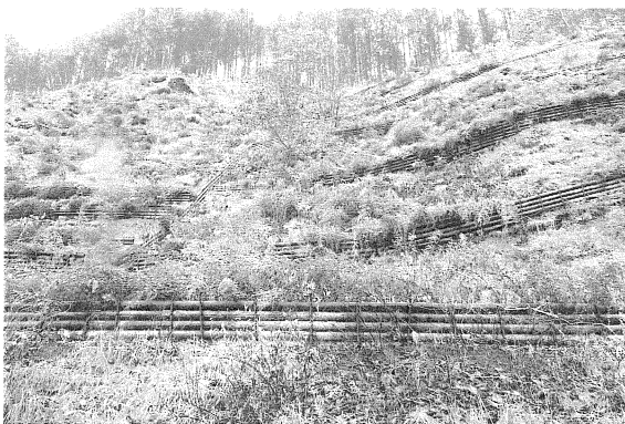
Nomugi Pass hillside work: example of the use of wood obtained by thinning trees
