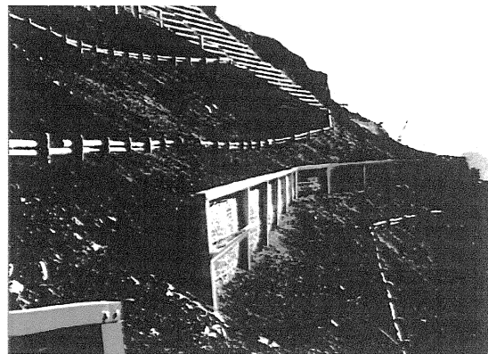
Onagi hillside work: on the earth retaining work, scoria that is easily moved by the wind etc. was firmly solidified.
