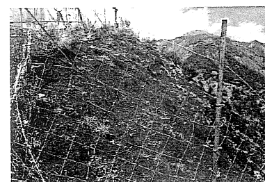
(Photo 3) Measure to prevent damage by deer: A protective net installed to prevent damage by Japanese serow and Japanese deer.
