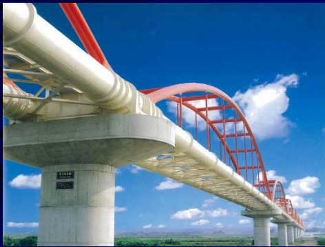
The longest water pipe bridge in Japan ( L = 1,100 meter )
