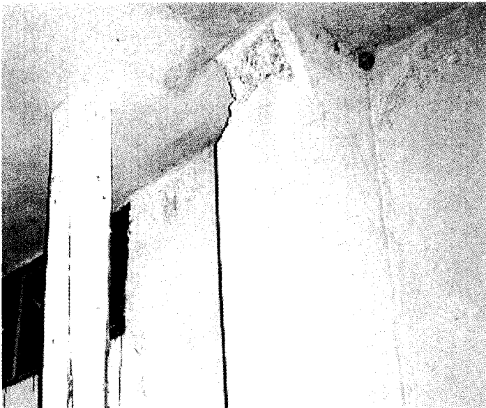
7) Big shear crack and spalling of cover concrete is observed at the top of column.
