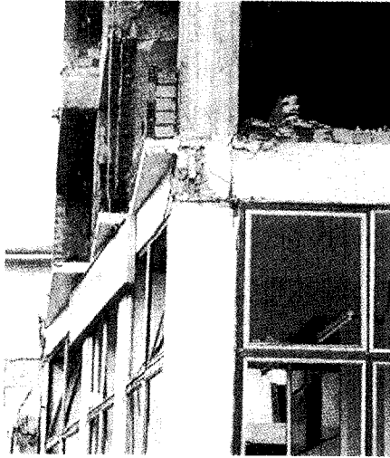
Diagonal shear cracks at the beam-column joint
