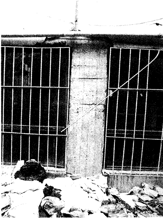
1) Mortar is separated and fallen down, and No shear cracks are observed.
