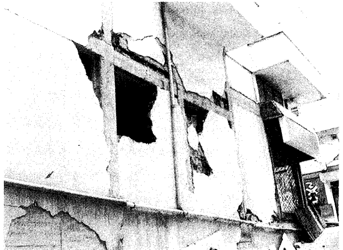
4) Rank C: Extensive cracks penetrated
