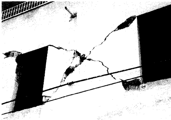
3) Rank C: Diagonal cracks observed
