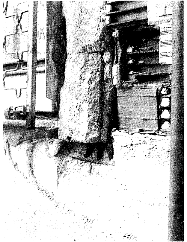
6) Damage is almost same as Fig.4.1.3.1 a). But the damage is heavier and there are cracks in core concrete.
