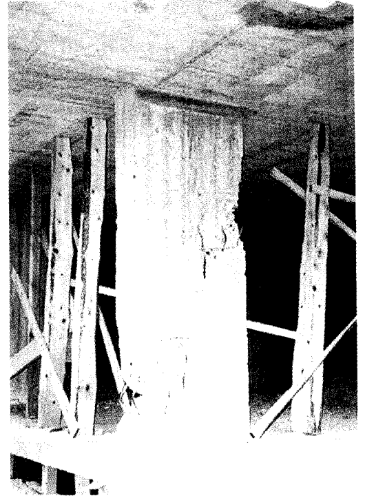
2) Buckling of reinforcing bars Crush of core concrete
