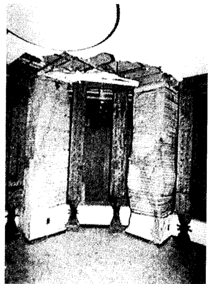
(5) Jacketing of damaged column with steel wires
