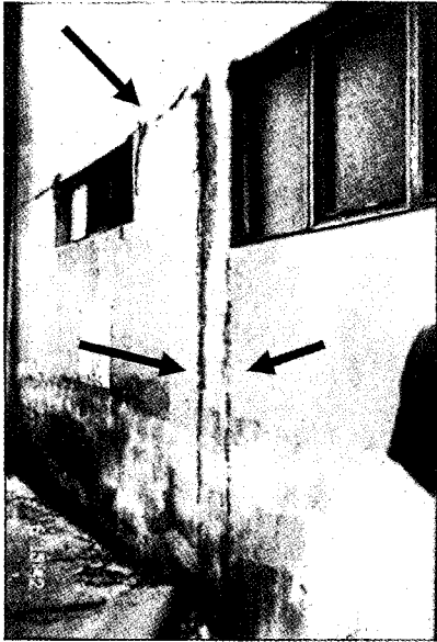
Cracks along interface between structural members (column and beam) and nonstructural wall are clearly observed.
