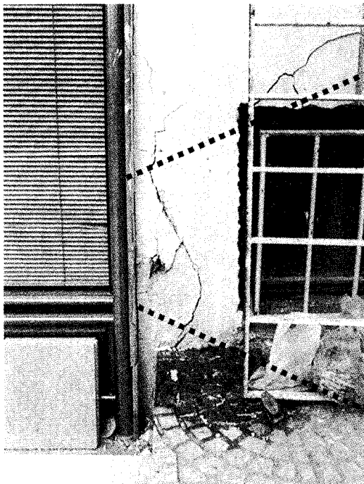
3) Big crack is observed on mortar. But take the mortar away, no crack is observed on the face of concrete.
