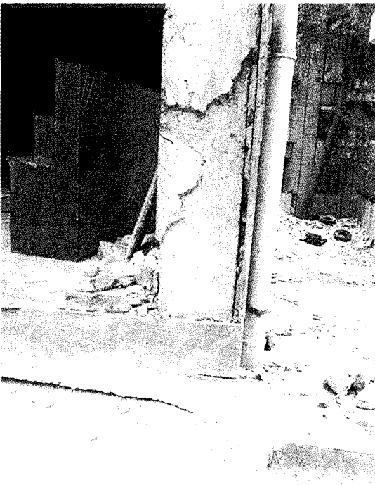
6) Corner cover concrete is spalled off. But shear cracks are not observed.
