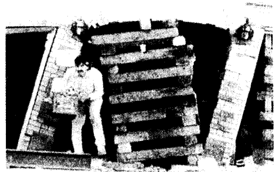
(2) Shoring with double crossed wooden layers
