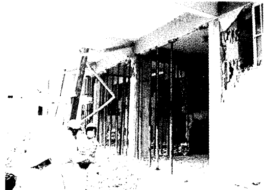
(4) Shoring with steel pipes or screw jacks around heavily damaged column
