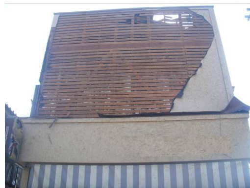
Photo 16 Wooden Building N
