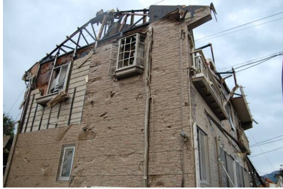
Photo17 Steel Framed Building A
