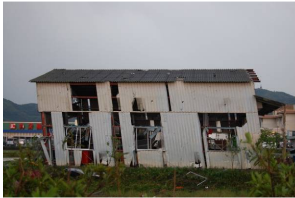
Photo 18 Steel Framed Building B
