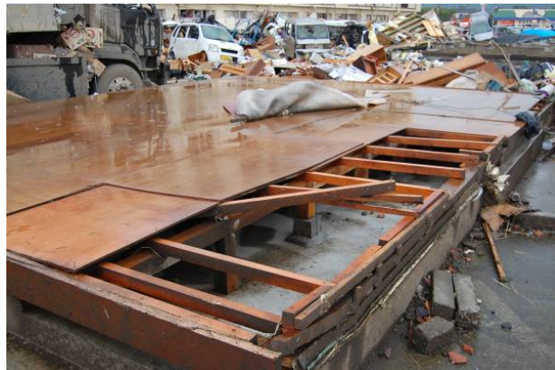
Photo 7 Wood House E
