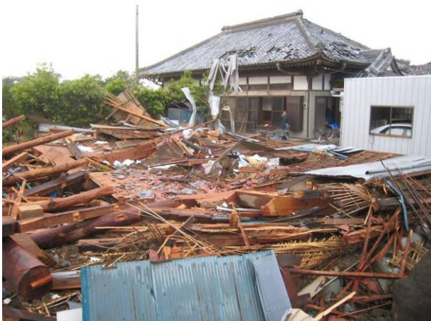
Photo 3 Wood construction B (this side, collapsed one)
