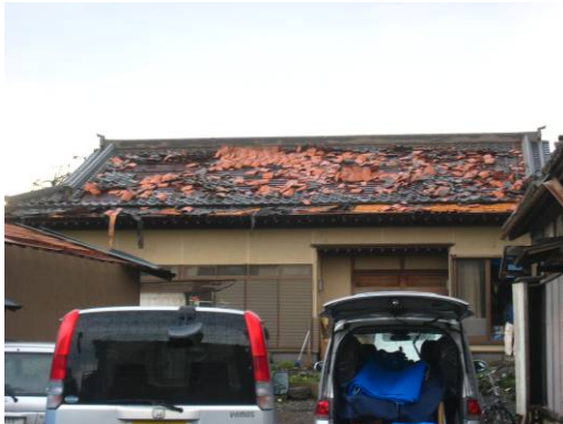
Photo 15 Wooden Building M
