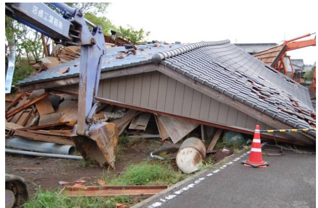
Photo 4 Wood construction C
