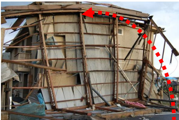
Photo 19 Steel Framed Building C
