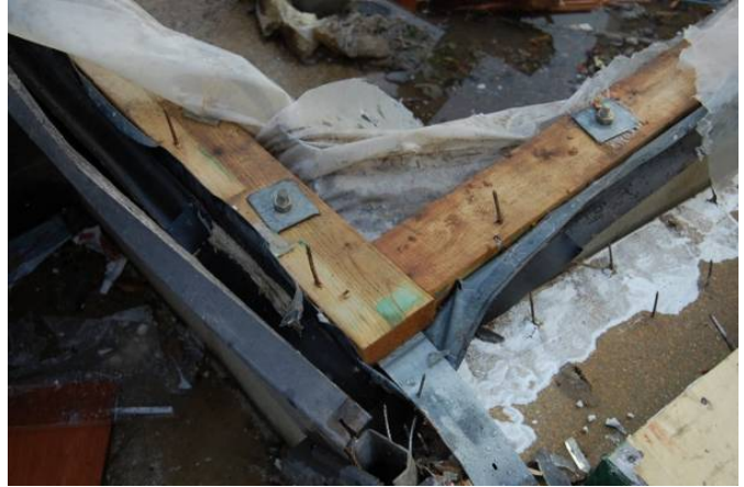
Photo 6 Remaining foundation of Wood House D
