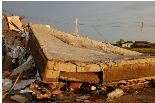
Photo 2 Turned mat foundation of Wood House B
