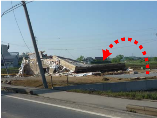
Photo 1 Wood House A
