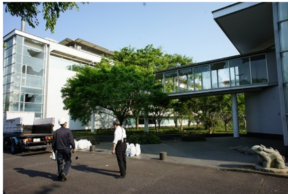
Photo 38 Broken window of a roofed passage
