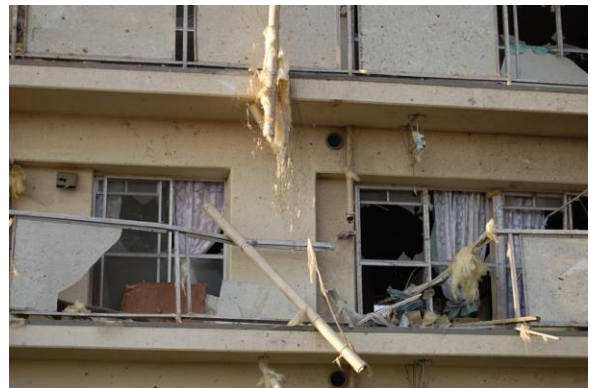
Photo 23 Windows and handrails 2
