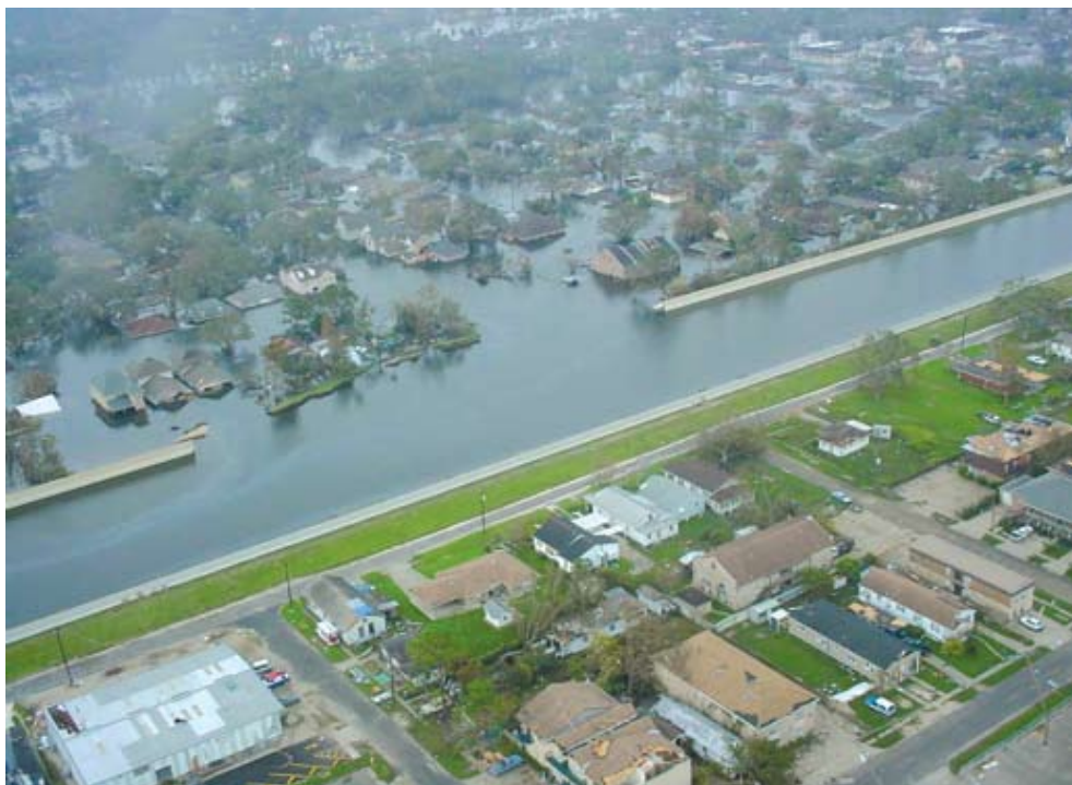
図-5.7 17th Street Canal の破堤
