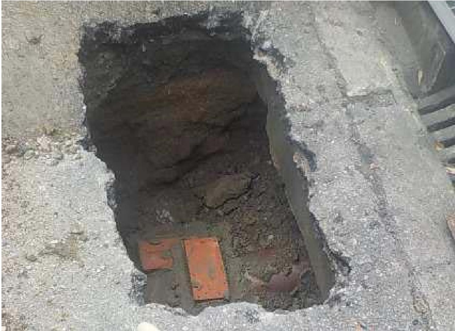
〇市：取付管、取付管接合部破損、長さ1.2×幅0.8×深さ0.7m
