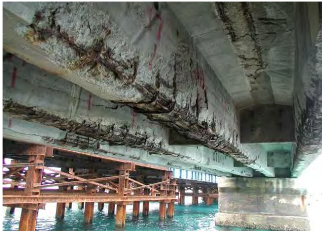
Chloride (Salt)-induced deterioration
