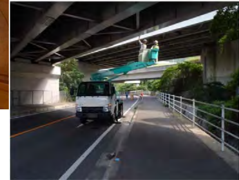
Close visual inspection of tunnel equipment and bridge
