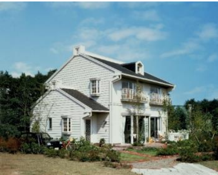
“House with a dormer window,” two-story detached house with light-gauge steel frames, produced by SEKISUI in 1983
