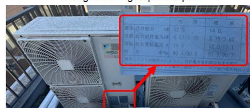
b) Confirmation of the capacity of air conditioning heat source (outdoor unit) on rooftop
