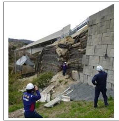
Photo-3 Investigation of mechanisms of disaster damage in the connecting section on the abutment back face
