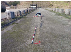
Cracks in top-end paved surface
