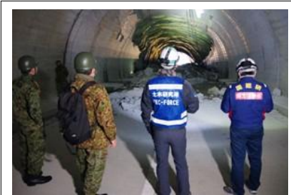
Photo-2 Investigation of the tunnel where the large-scale liner spalling occurred
