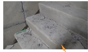
Deformation of horizontal joint parts (dam body)
