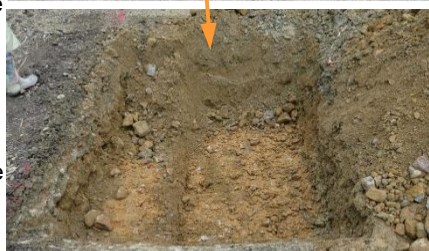
Excavation survey at cracked areas on dam's top-end paved surface (no damage in the dam body)
