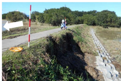
Photo-1 Erosion of inner slope at the area where the risk management type hardware measures have been taken
