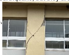
Shear destruction of a column
