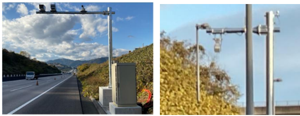
(a) Vehicle detection sensor (b) Information provision facility Fig.-4 Experimental devices for the provision of merging support information (near the Hamamatsu SA on the Shin-Tomei Expressway)
