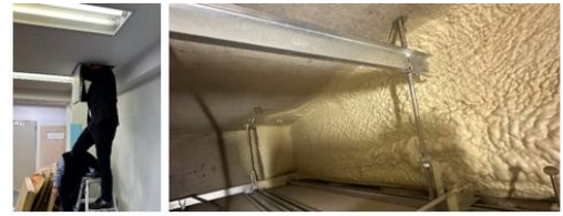
a) Confirmation of whether thermal insulation is performed through a ceiling inspection port
