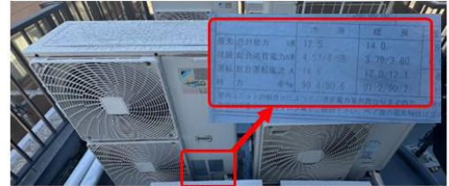
b) Confirmation of the capacity of air conditioning heat source (outdoor unit) on rooftop
