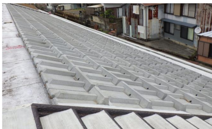
Photo-2 Example of highly resistant river embankment
