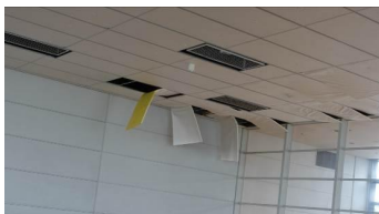
Ceiling collapse damage
