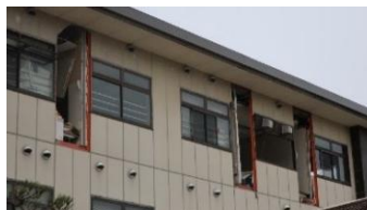
Exterior wall detachment damage
