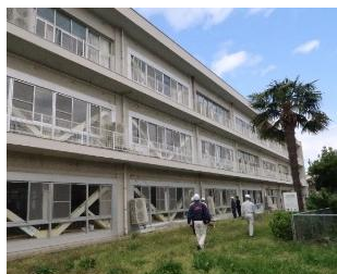
Exterior wall detachment damage
