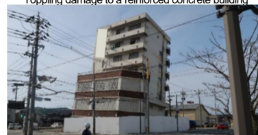
Inclination damage to a reinforced concrete building
