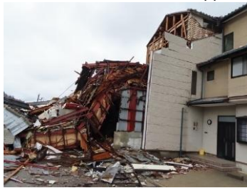
Collapse of 2nd and 3rd floors of a steel frame building
