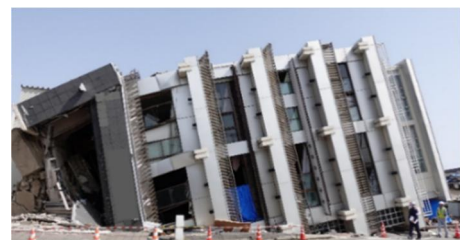
Toppling damage to a reinforced concrete building
