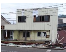
Layered collapse of the 1st floor of a steel frame building
