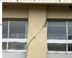
Shear destruction of a column
