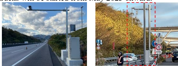
Figure-1 Experimental equipment for the provision of information on merging support (left: vehicle detection sensor, right: information provision facility)
