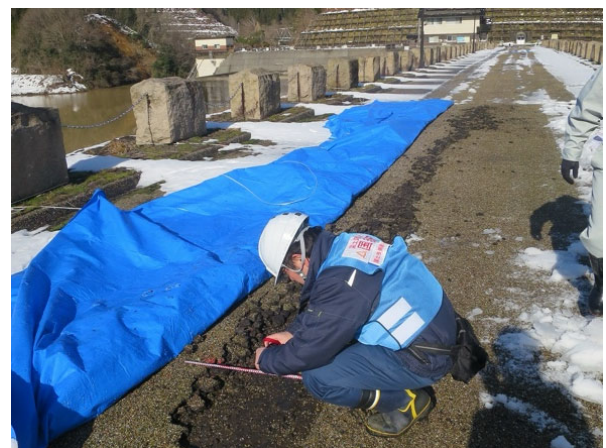
Photo-4 Survey of a dam damaged by the Noto Peninsula Earthquake
