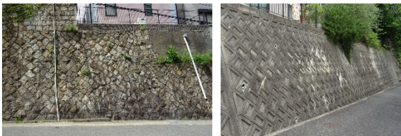
Photo: Example of a housing site with retaining wall construction
