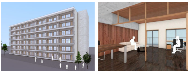
Fig. 1: Example for the prototype of wood mixed structure: Wooden walls and floors with RC frame on each floor (Left: Exterior, Right: Interior)
