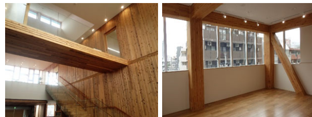
Photo 1: Design to show the timber as it is, which is the main structural member (left: medium-rise large-scale building, right: high-rise building)
