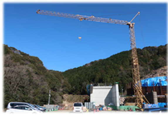
Fig. 3. Fixed horizontal jib crane
