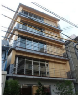
Photo 2: Example of "vertical wood-mixed structure": Mixed structure where the structure differs depending on floors. In this case, the first floor is RC and the second to fifth floors are wood (CLT).
