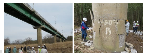
On-site investigation of Edano Bridge
