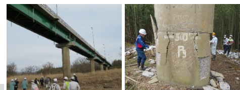
On-site investigation of Edano Bridge
