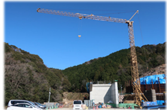
Fig. 3. Fixed horizontal jib crane
