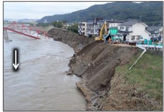
Photo 4 Levee collapse at 104 kp on the left bank of the Chikuma River Situation of damage (Oct. 15)
