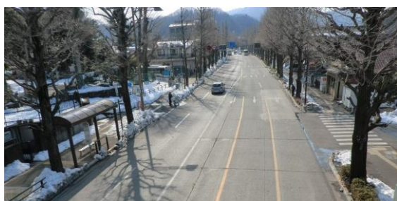
Photo 1. Concrete pavement on National Highway No. 20 in Hachioji City in Tokyo (In service since 1957. Photo taken in February 2014)
