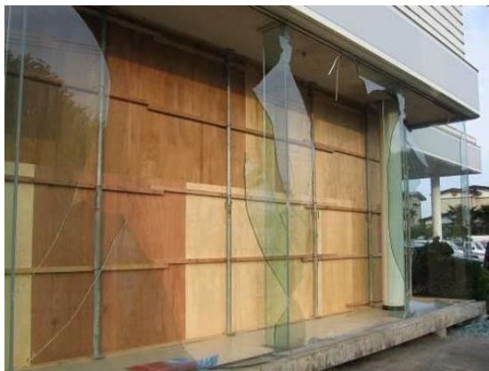
Photo 1: Damaged glass screen by earthquake after its damage
