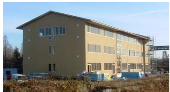
Photo 1. The Experimental Three-story Wooden School Building
