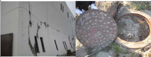
Figure 1. View of Damaged Sewage Facilities
