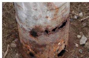
Photo 1. Column Base Corrosion Covered by Paving
