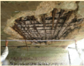
Bridge with internal steel rods exposed Riverbank protection with cracking
