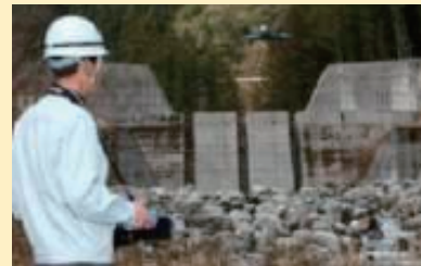
Inspection of facilities related to Sabo by utilizing drones
