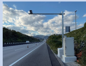
Equipments for field operational test (left: vehicle detection sensor, right: information provision unit)
