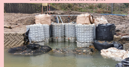
Water intake facility in a water purification plant rehabilitated during the emergency (Suzu City)
