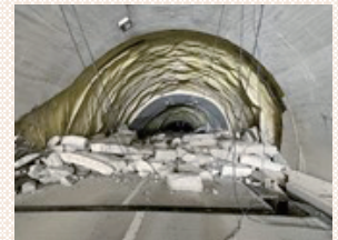
Example of tunnel lining collapse in the Noto Peninsula Earthquake
