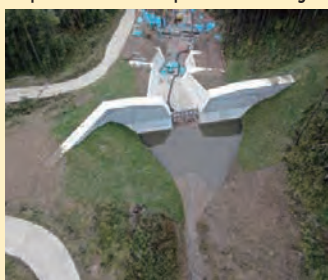
Construction of a Sabo dam with high capture capacity of sediment and driftwood trapping performance (Suzaka City, Nagano Prefecture)
