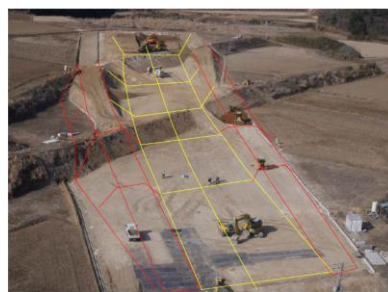
Construction site without need for finishing stakes (optimization of construction/construction management)
