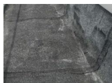
Swelling of waterproof layer; removal of waterproof layer required for long service life
