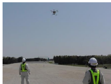
Earthwork measurement by means of UAV (optimization of construction/construction management)
