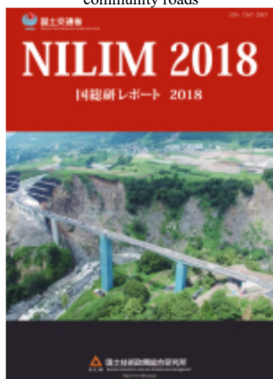
Restoration of a road bridge (Minamiaso Village, Kumamoto Prefecture) damaged by the Kumamoto earthquakes (opened in August 2017)
