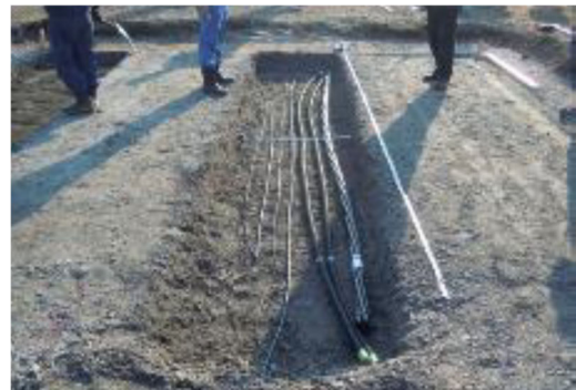
Figure 8: Construction experiment on shallow burial of cable
