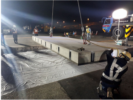
Figure-5 Construction of high-strength RC precast pavement
