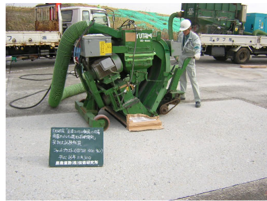
Figure-6 Existing pavement surface treatment by shot blasting
