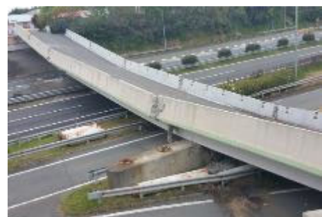
Photo 4: Damage to bridge with locking piers (Kumamoto Earthquake)
