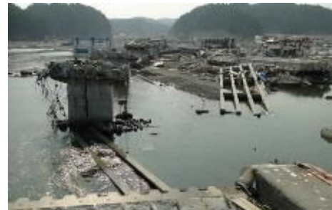
Photo 2: Damage to bridges damaged by the tsunami (Tohoku Earthquake out at Pacific Ocean)
