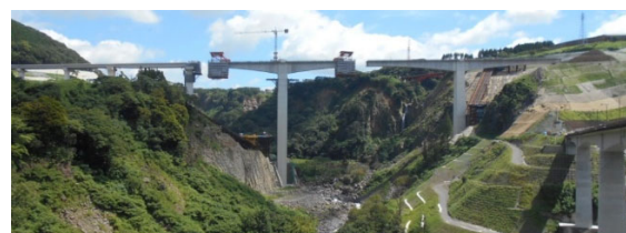
Figure 6 The New Aso Bridge where the bridge girders remain without falling off even when the ends of the girders are not on the bridge piers (under construction) (Photo provided by the Kumamoto Reconstruction Project Office)
