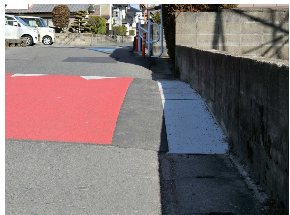
側溝上も併せて嵩上げ
