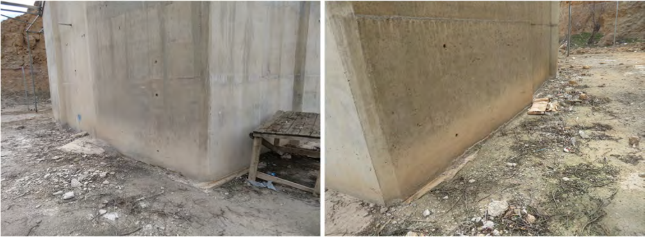
Figure 2.4-19. Base of east-side pier
