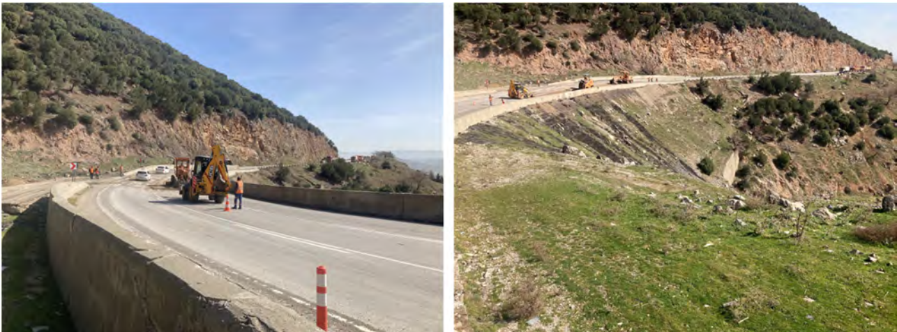
Figure 2.3-17. Repair of National Highway D400 near Atatürk viaduct
