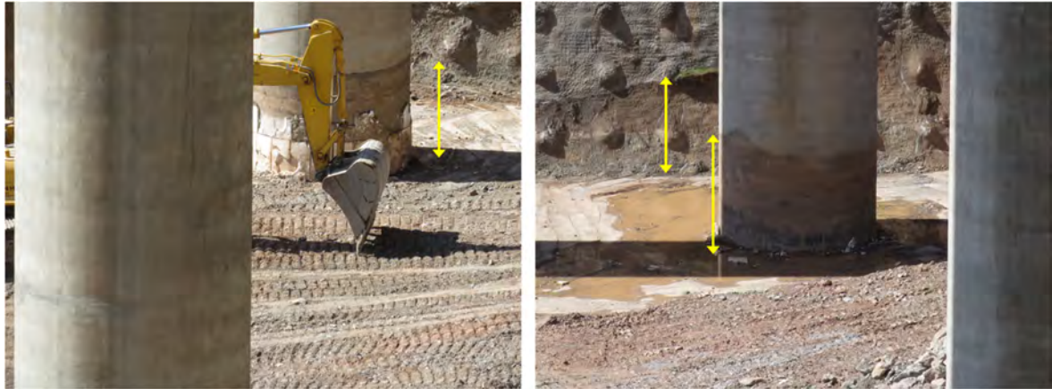
Figure 2.3-27. Grounds surrounding bridge piers
