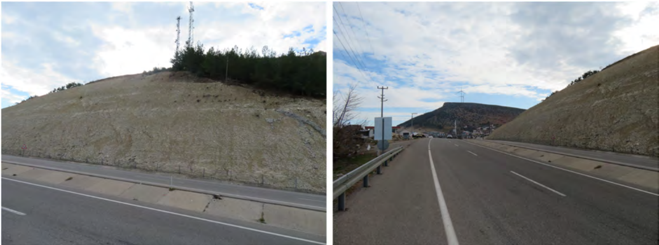
Figure 2.5-6. Example of cut slopes
