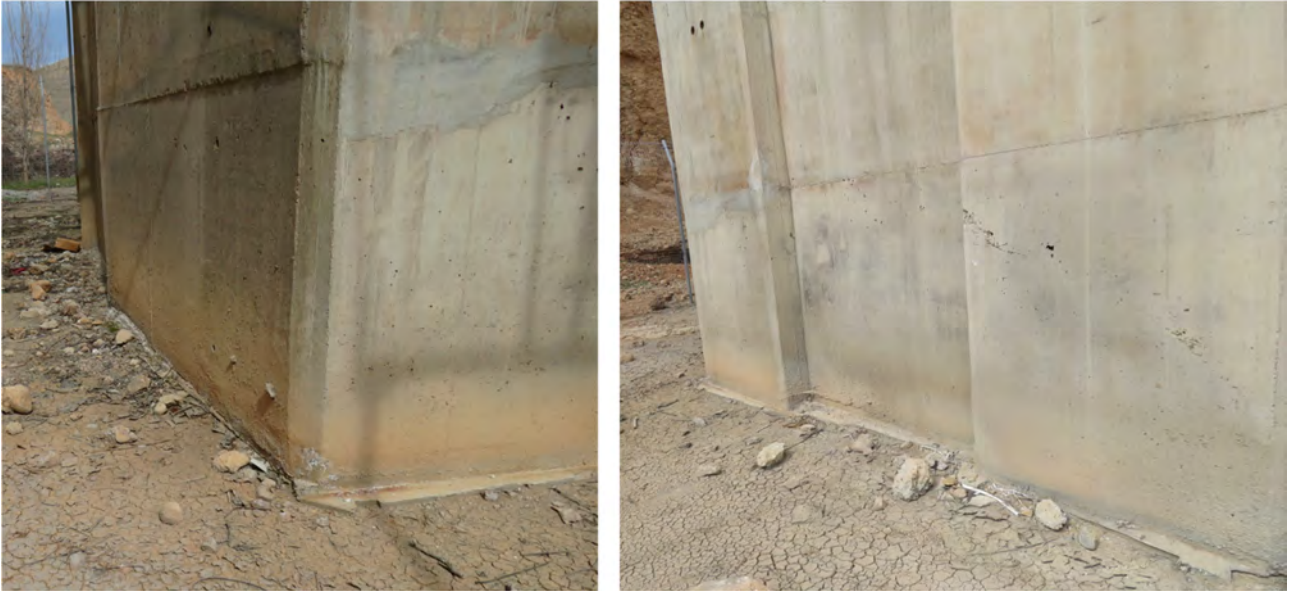
Figure 2.4-21. Base of west-side pier
