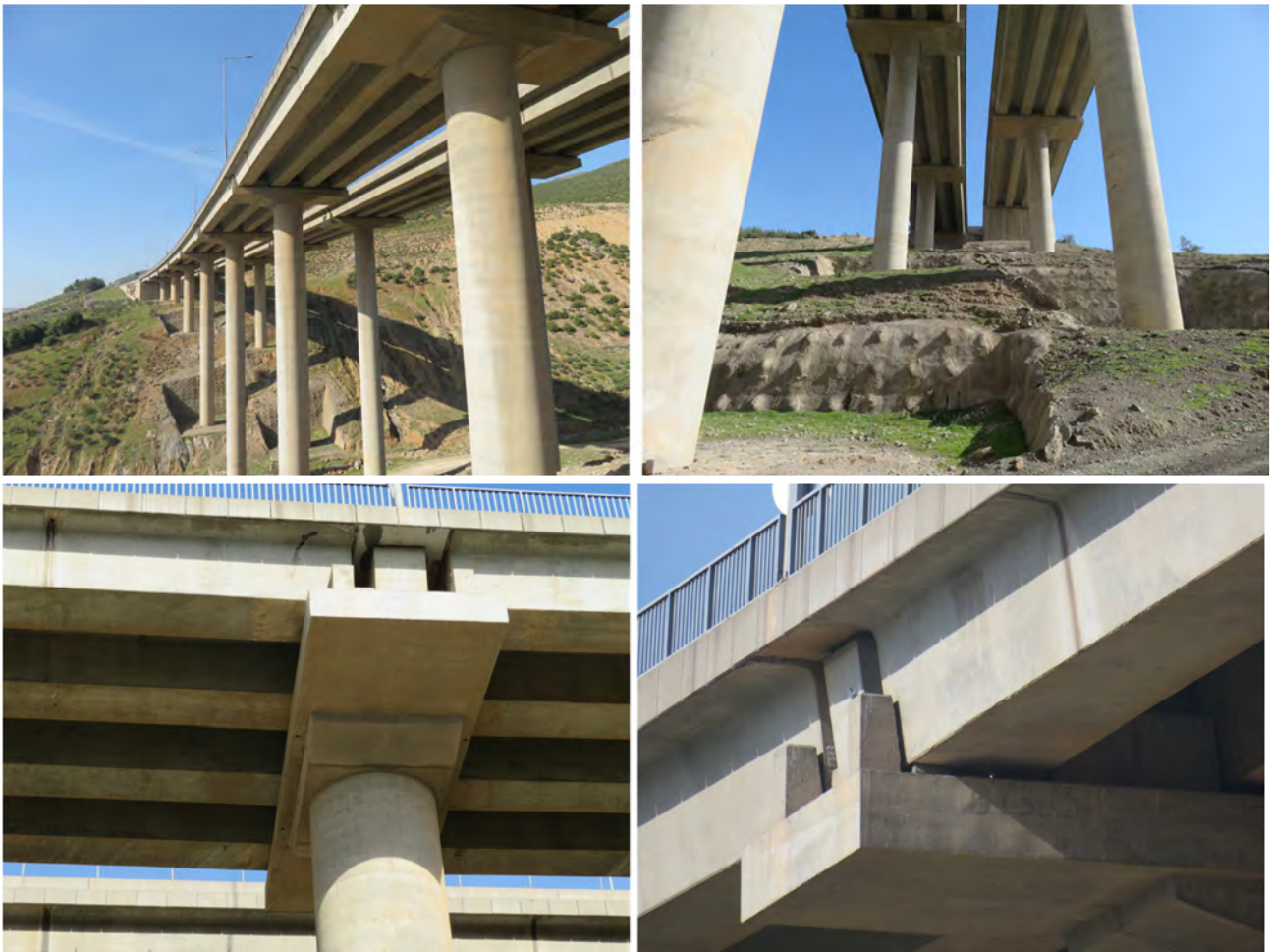
Figure 2.3-3. Başpınar viaduct on O52
