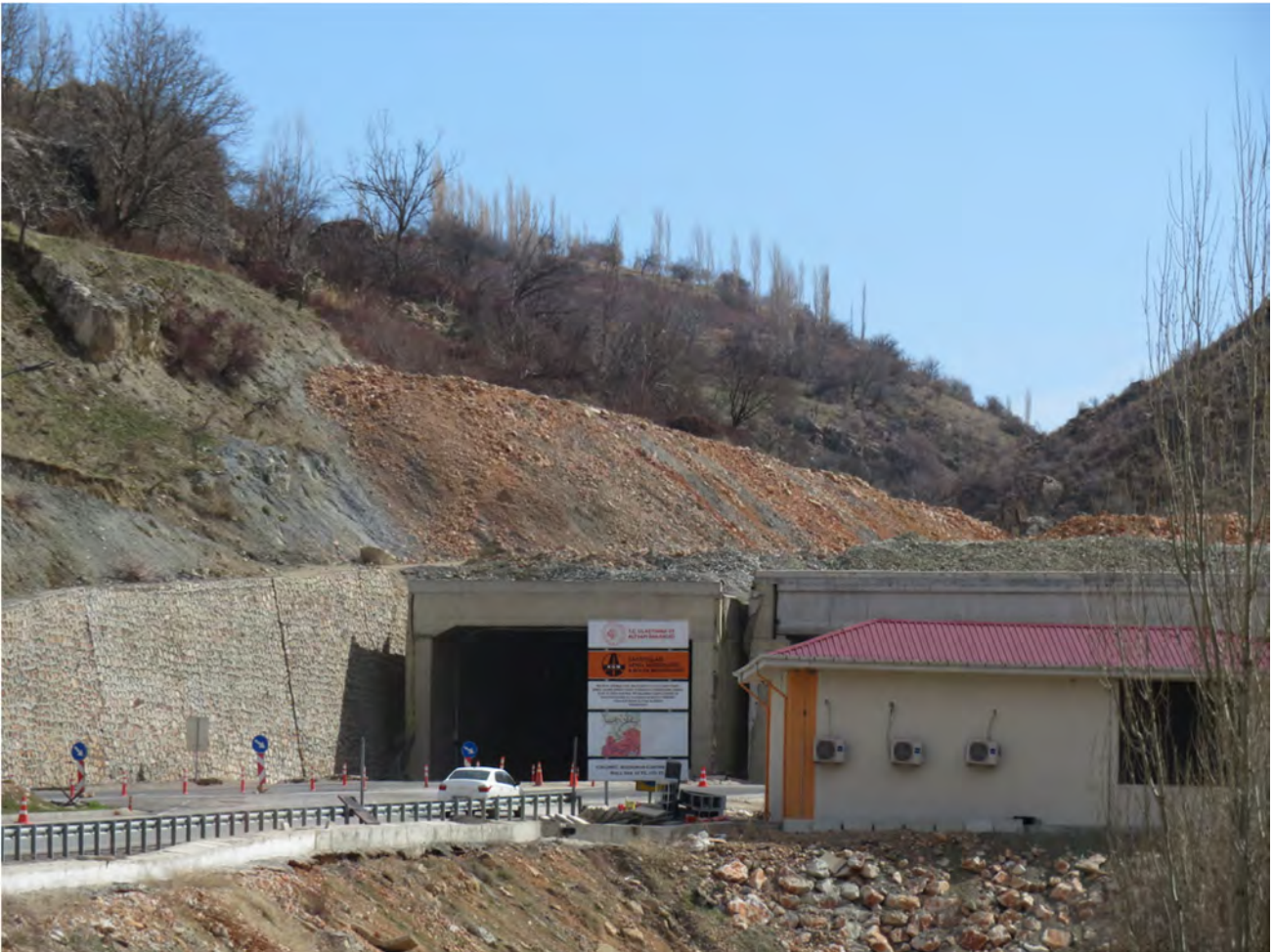
Figure 2.4-10. Rock shed adjacent to Erkenek tunnel
