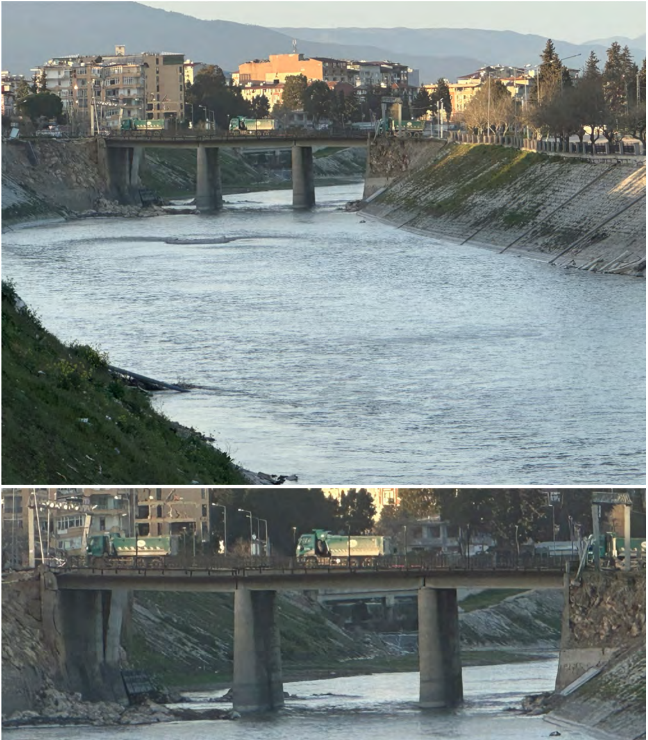
Figure 2.1-17. Photos of a bridge taken from Bridge #4
