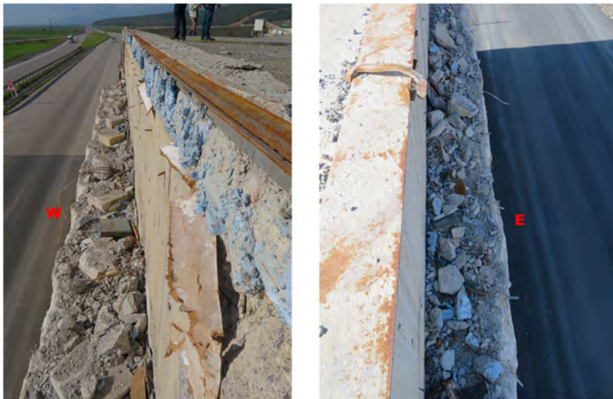
Figure 2.2-6. Comparison of bridge seatings in west and east-side abutments
