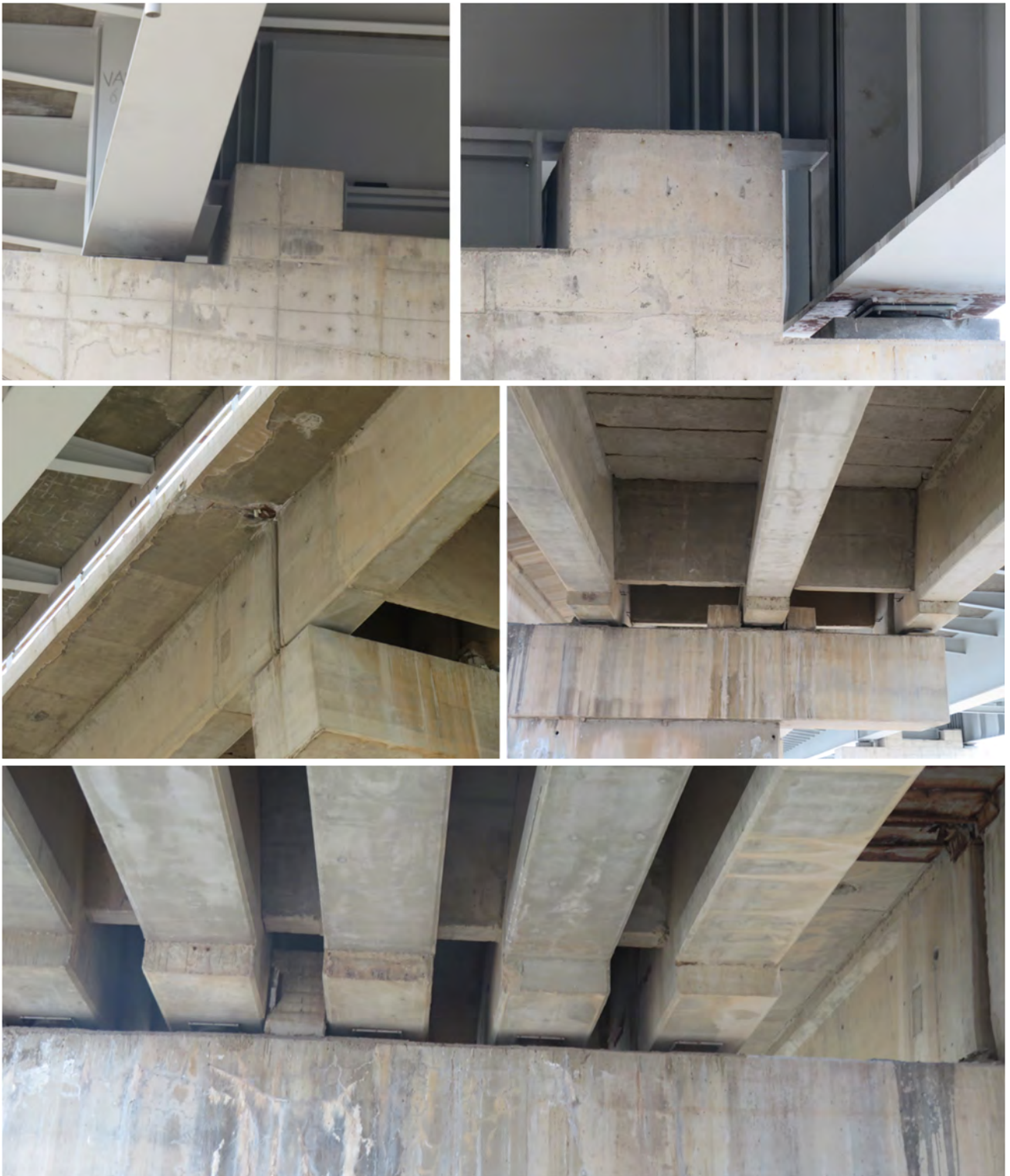
Figure 2.4-38. Shear keys on pier caps
