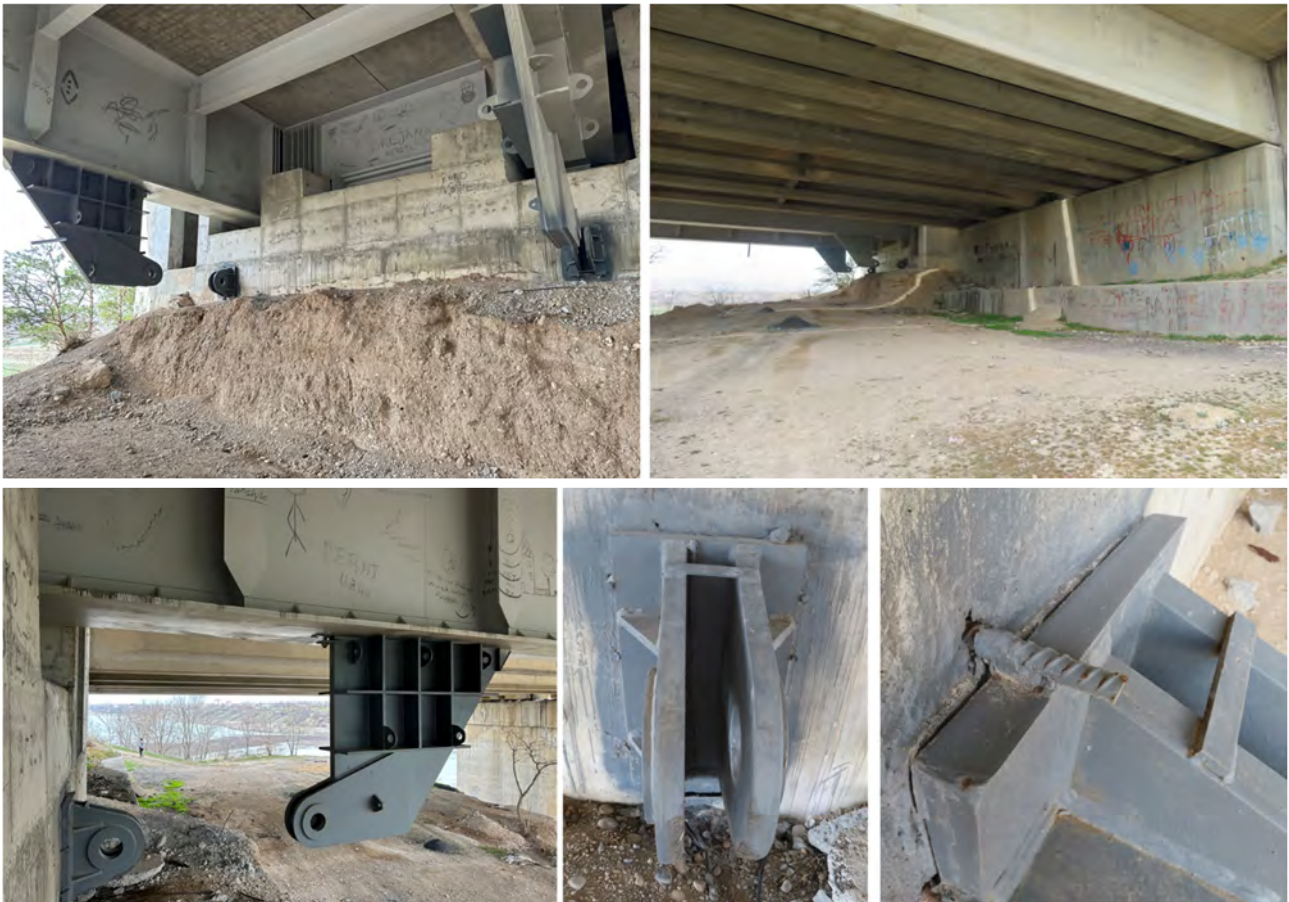
Figure 2.4-35. Close-up views of north-side abutments
