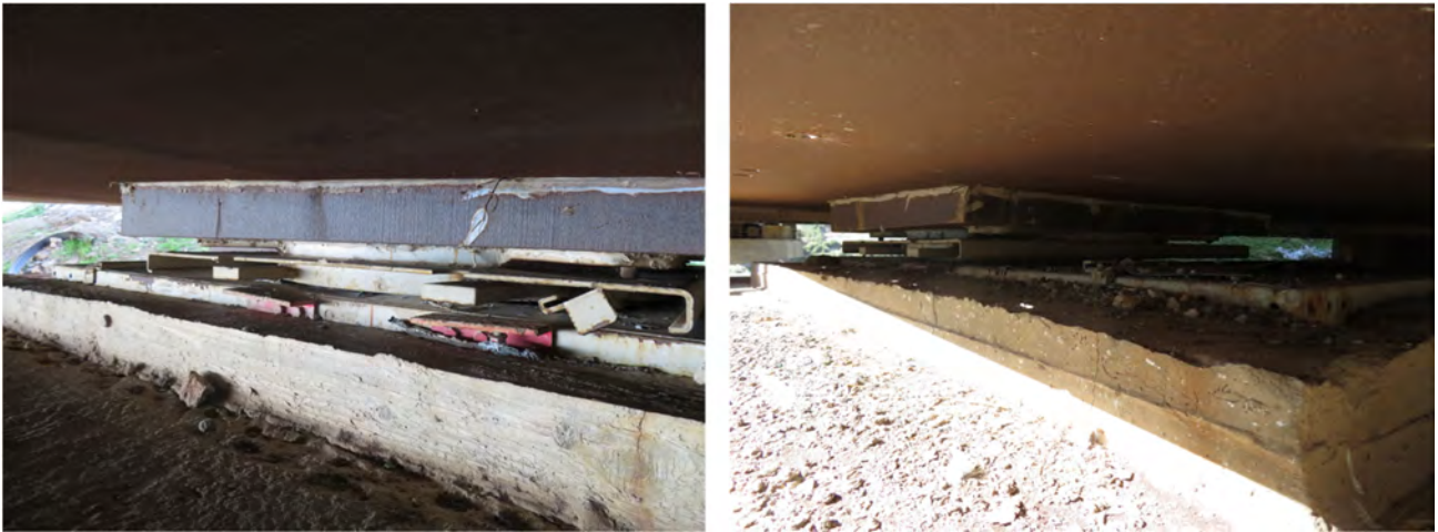
Figure 2.3-12. Bearing support on abutment
