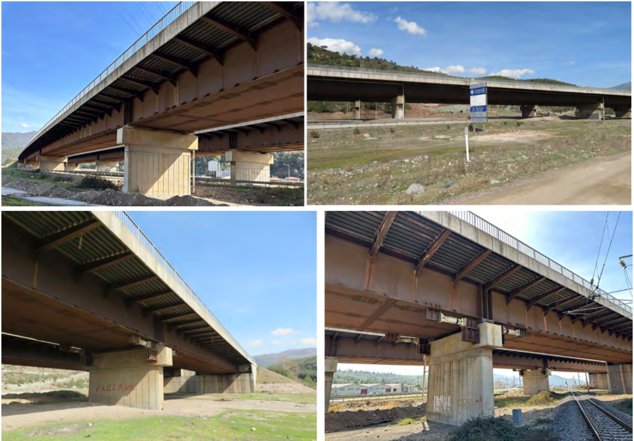
Figure 2.3-42. Vecdi Diker viaduct on O52
