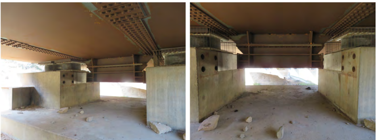
Figure 2.3-35. Horizontal displacement restrainer of girder and concrete blocks on column next to Gaziantep-side abutment
