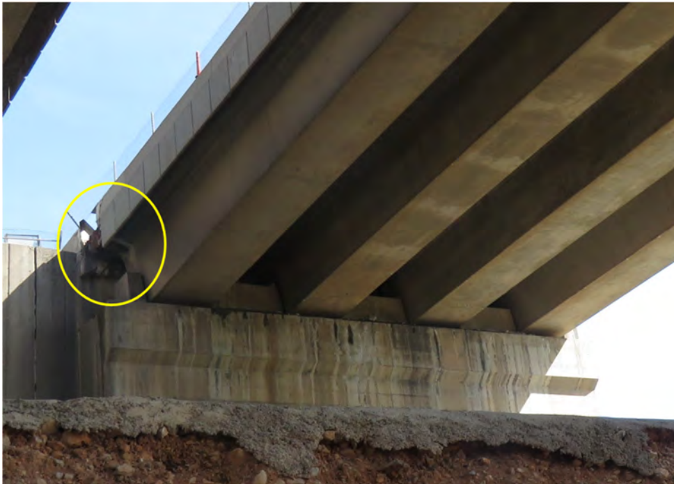
Figure 2.3-22. Gaziantep-side abutment on in-service side of bridge
