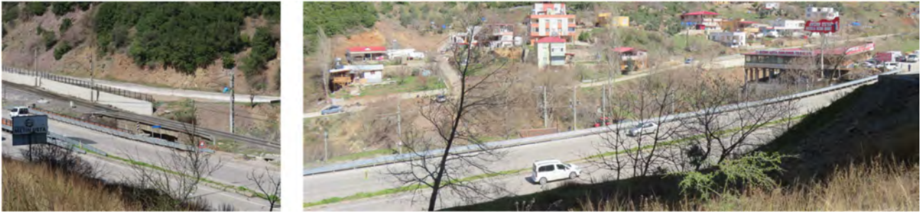
Figure 2.3-40. Roads and buildings around viaduct
