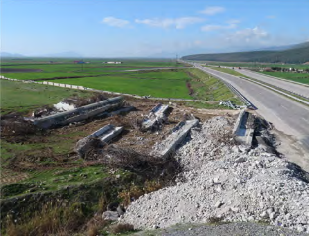
Figure 2.2-3. Abutments and removed girders
