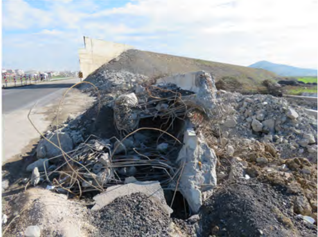
Figure 2.2-3. Abutments and removed girders
