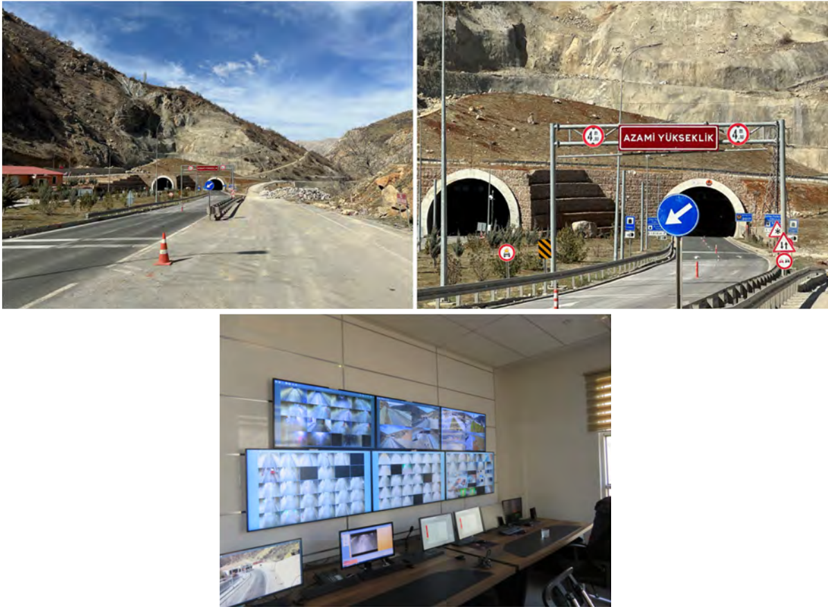
Figure 2.4-7. Erkenek tunnel on D850 and operation office
