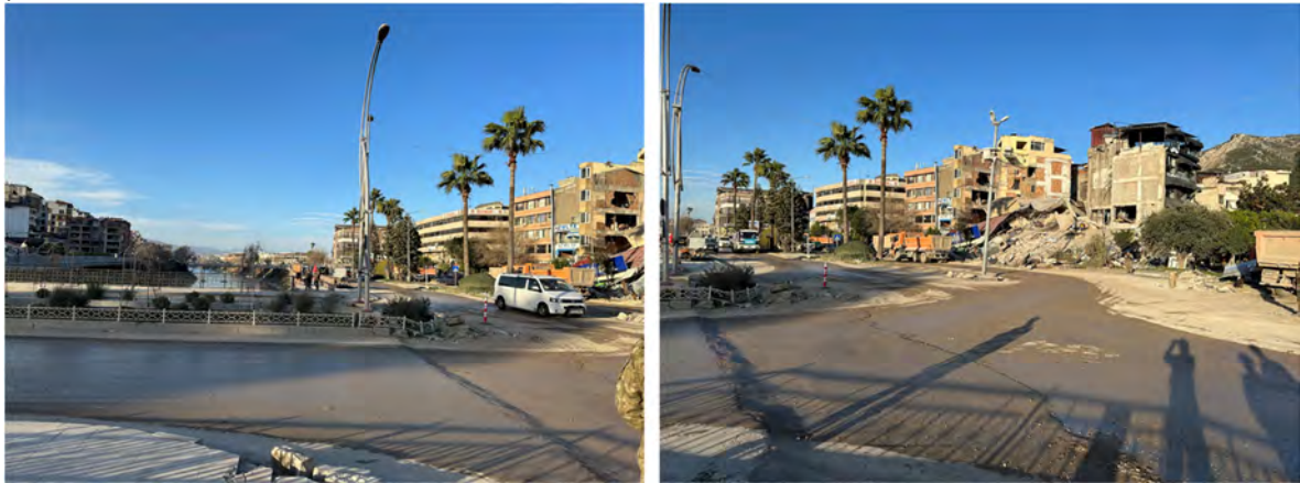
Figure 2.1-11. Approaches to Bridge #3
