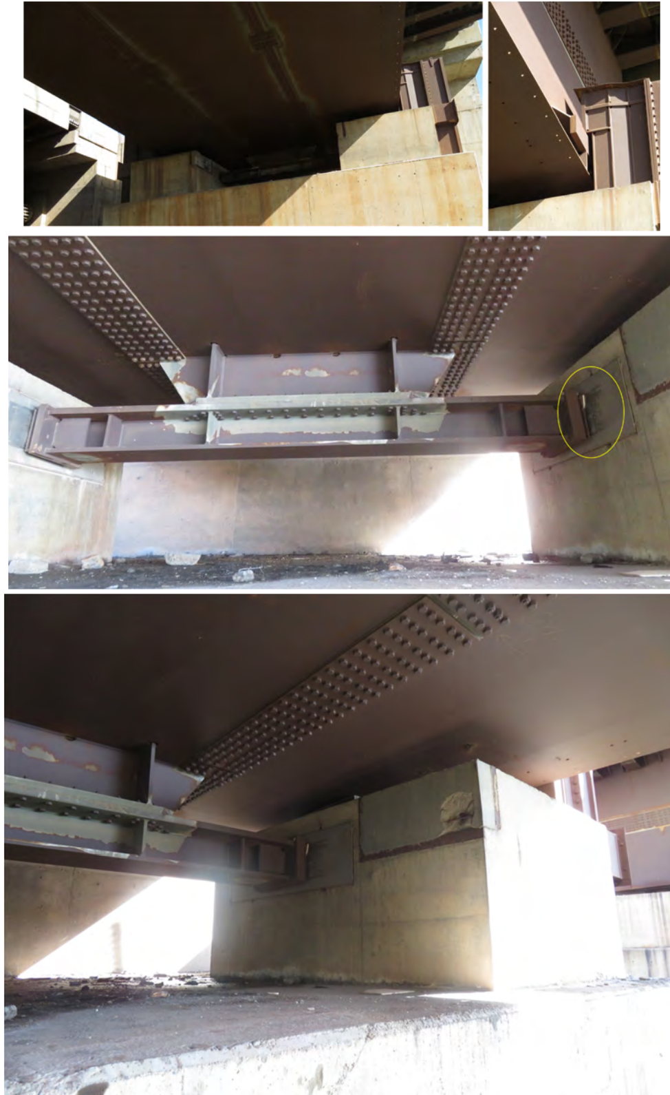
Figure 2.3-11. Lateral stopper below lower flange of box girder
