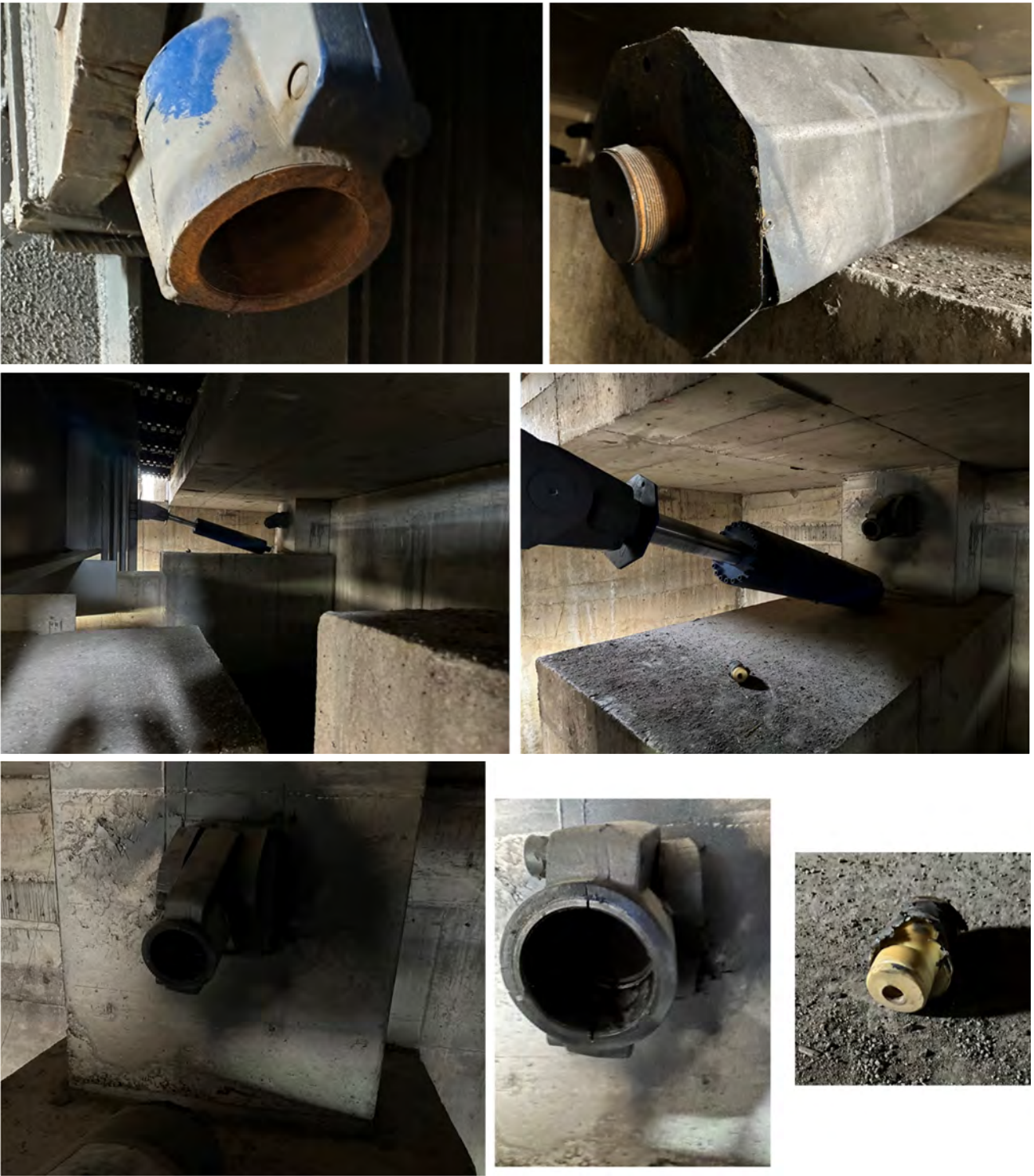
Figure 2.4-27. Connection parts of dampers
