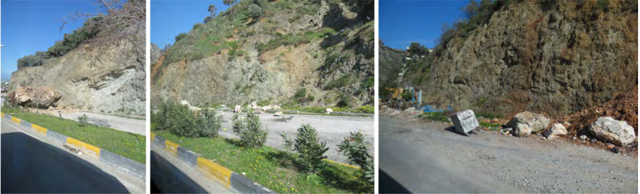
Figure 2.5-2. Rockfalls in suburban Antakya
