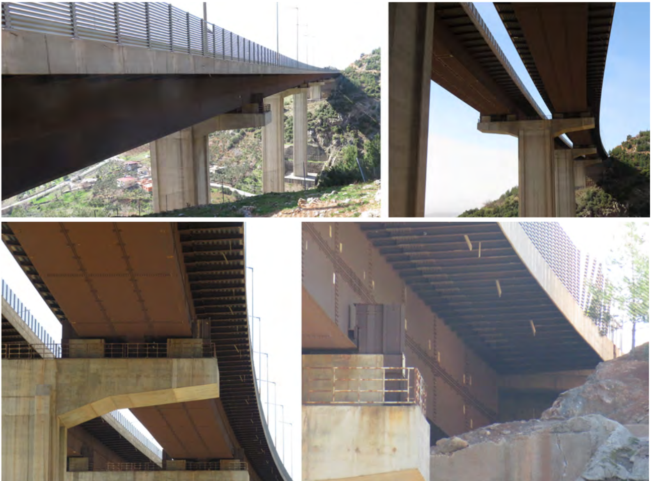
Figure 2.3-8. Turgut Özal viaduct on O52
