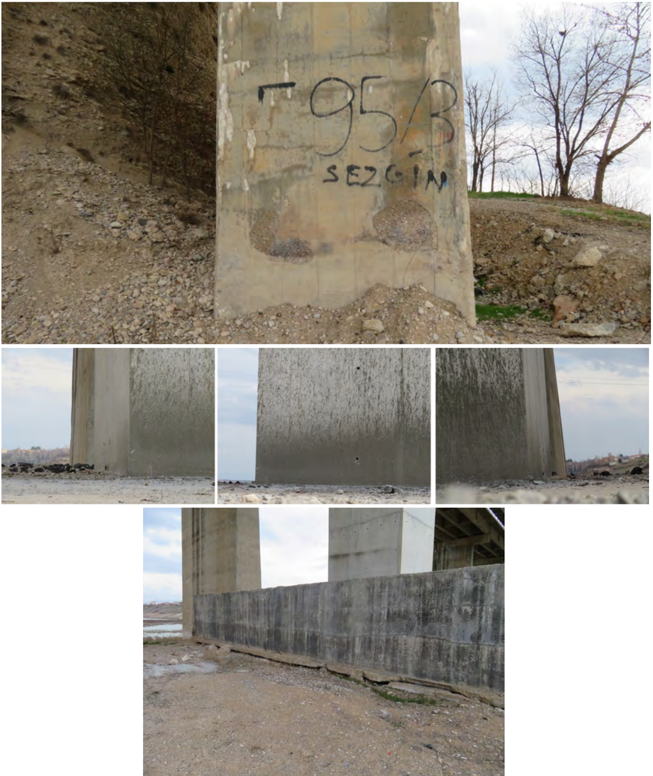
Figure 2.4-39. Bases of some piers and surrounding ground surface
