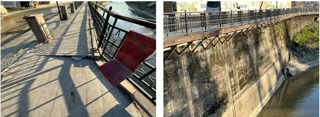
Figure 2.1-12. Pedestrian deck along river near Bridge #3
