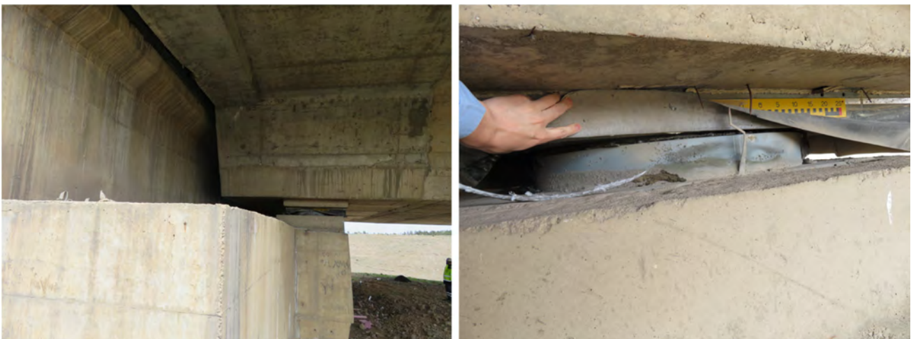
Figure 2.4-17. Bearings and their covers
