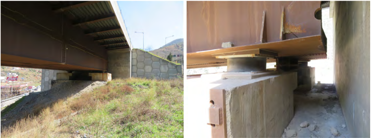
Figure 2.3-36. Superstructure and Gaziantep-side abutment on D400-side bridge
