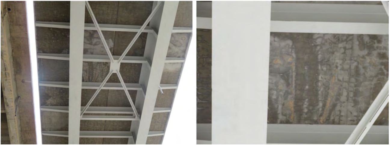
Figure 2.4-40. Deck slabs of new bridge
