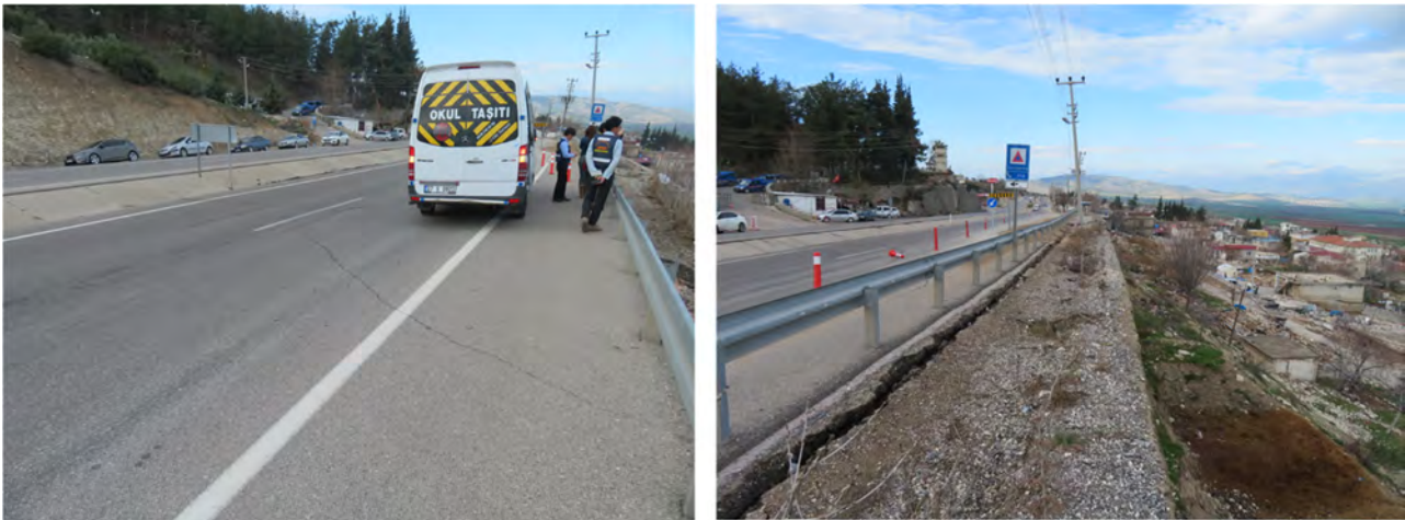
Figure 2.5-4. Traffic restriction on shoulder
