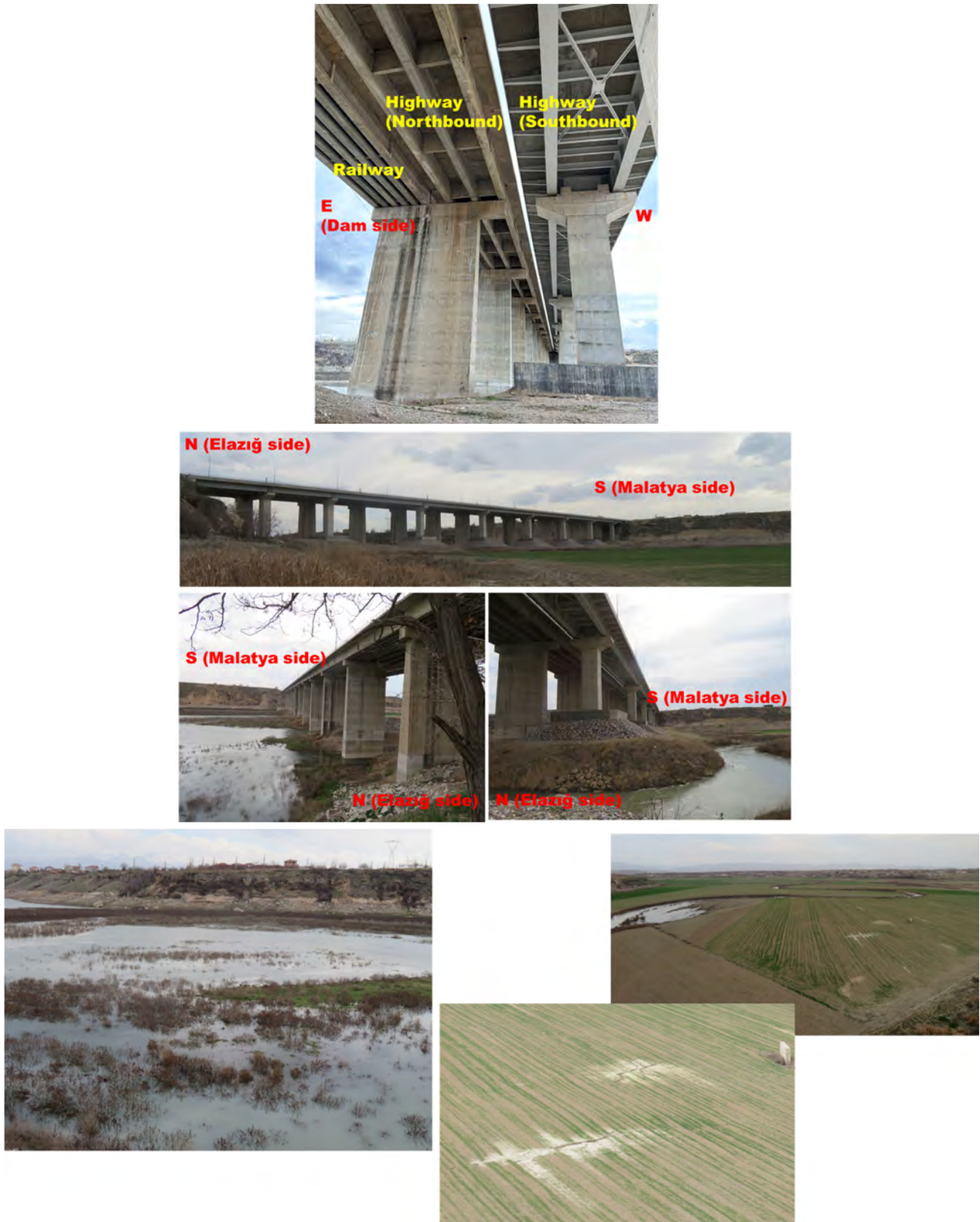
Figure 2.4-24. Tohma bridge on D875 Malatya/Keban highway
