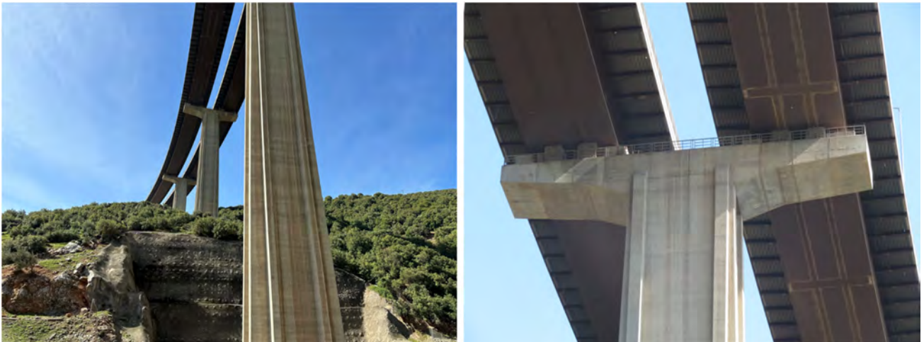
Figure 2.3-15. Atatürk viaduct on motorway O52
