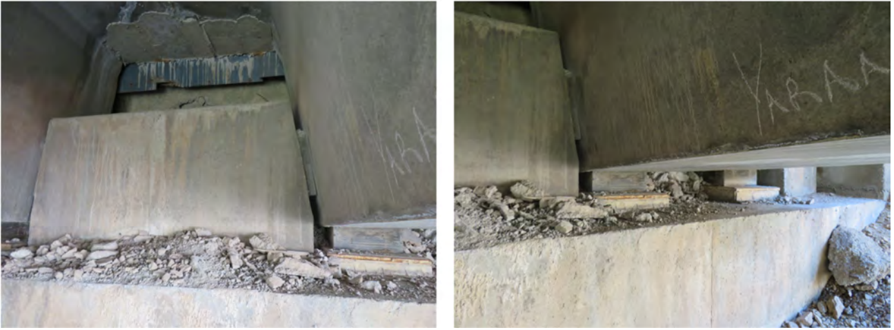
Figure 2.3-38. Tub girders, shear keys, and bearings
