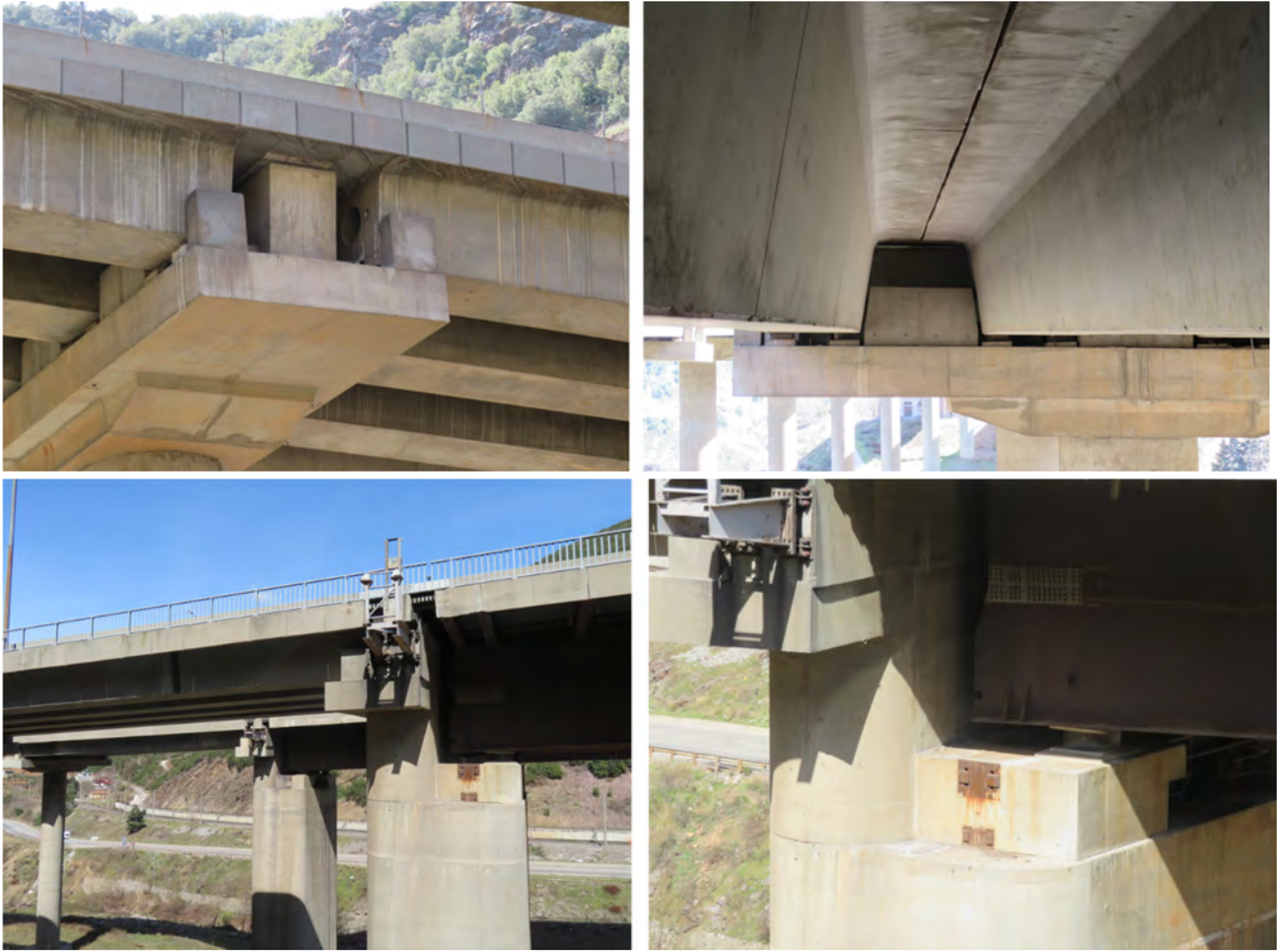
Figure 2.3-32. Girder-column connections
