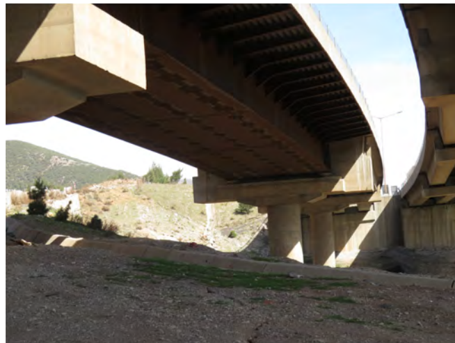
Figure 2.3-19. Nurdağı viaduct on O52
