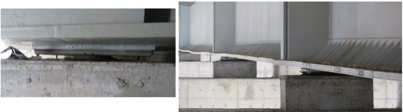
Figure 2.4-37. Bearings on piers of new bridge
