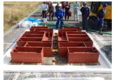
⑤ 鋼製山留設置
