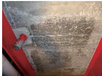
(e) 床版下面の遊離石灰
