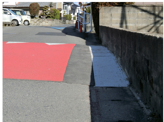
側溝上も併せて嵩上げ
